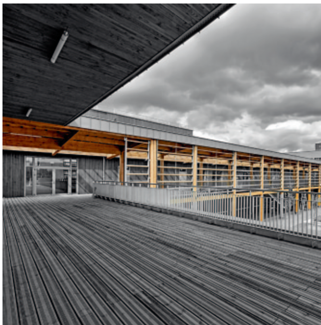
Gergovie high school, a building with a minimal carbon impact, Clermont-Ferrand (Puy-de-Dôme) © Eiffage/Joël Damase
