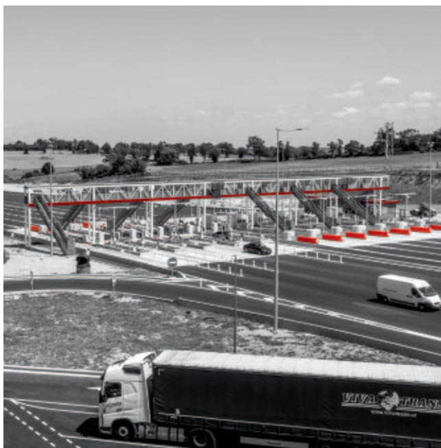
Free-flow toll station on the A79 motorway, Digoin (Saône-et-Loire) © Eiffage
