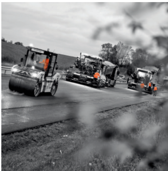
Installation of Biophalt® plant-based asphalt, A40 motorway Vonnas-Mâcon (Ain) © APRR
