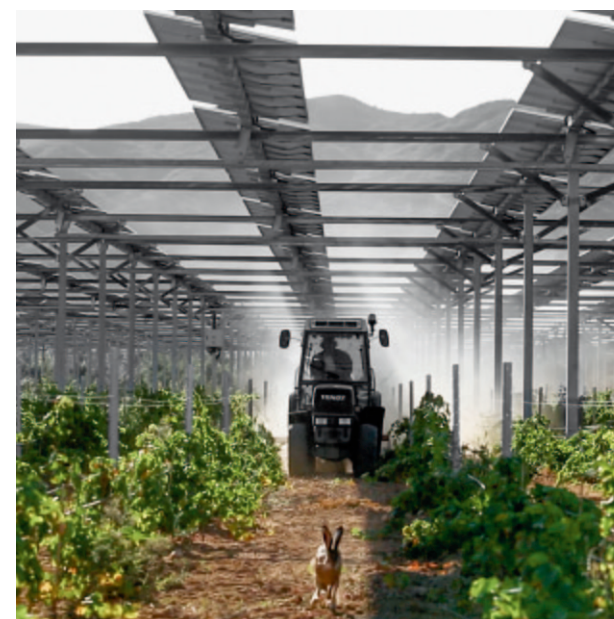
Photovoltaic panels installed above the vines, Tresserre (Pyrénées Orientales) © Sun'Agri
