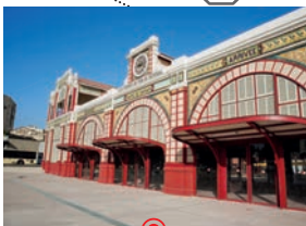
— Regional railway Dakar (Senegal) Design-and-build contract for a regional railway line linking central Dakar to Blaise-Diagne international airport (AIBD).
