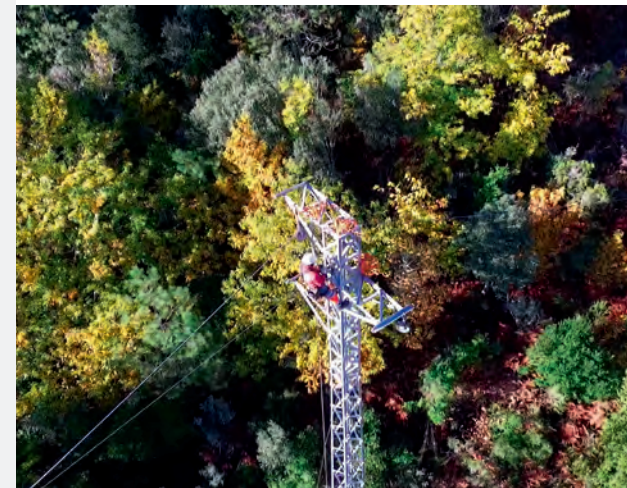
Spain — Maintenance of Iberdrola power lines
