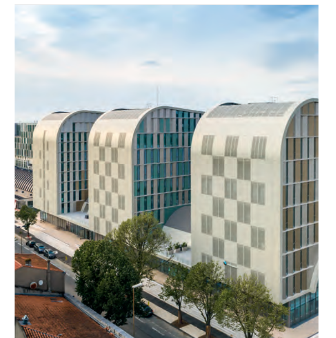
Bordeaux (France) — Eiffage Immobilier delivered Halle Boca, a mixed-use building spanning 23,500 m 2 in the heart of the Euratlantique district.
