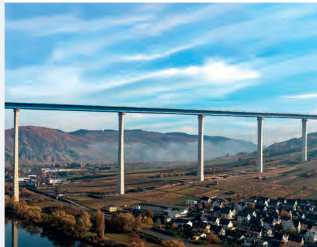
Rhineland-Palatinate (Germany) — The Hochmosel bridge
