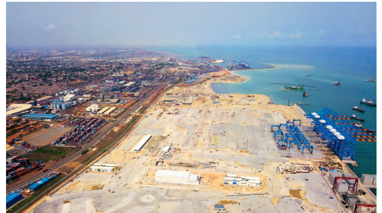
Tema (Ghana) — Eiffage designing and building a 97.6-hectare port platform.
