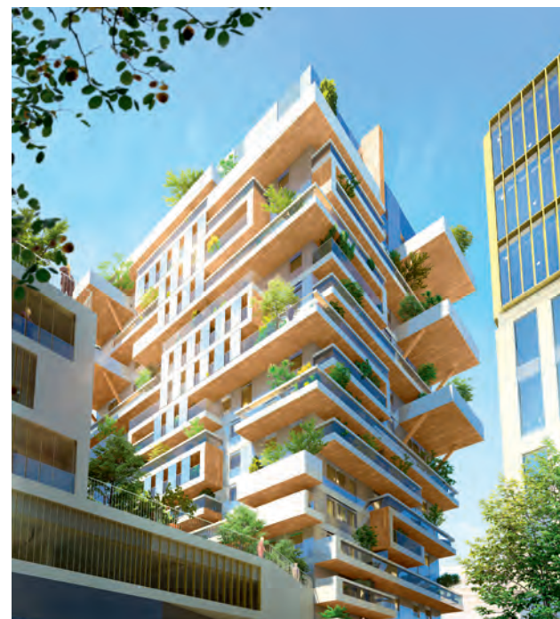
Bordeaux (France) — Apartments in the Hypérion tower went on sale in late 2018, and work started at the beginning of 2019. Hypérion will be France’s tallest residential building with a wooden frame and façades when it is delivered in 2021.
