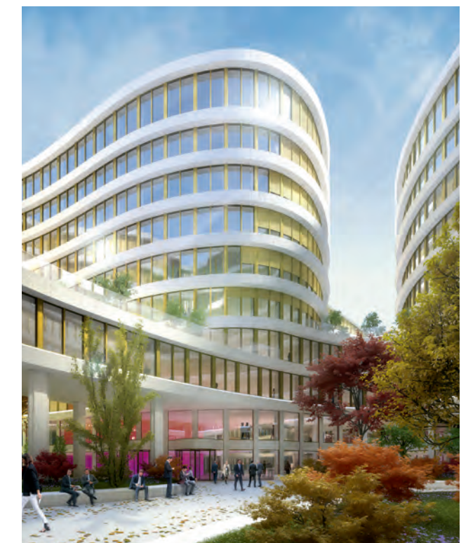
Brussels (Belgium) — Eiffage is building BNP Paribas Fortis’ new headquarters.
