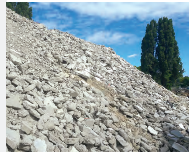
With selective deconstruction, we can separate and sort the various elements demolished in situ so that they can be recycled or reused.
