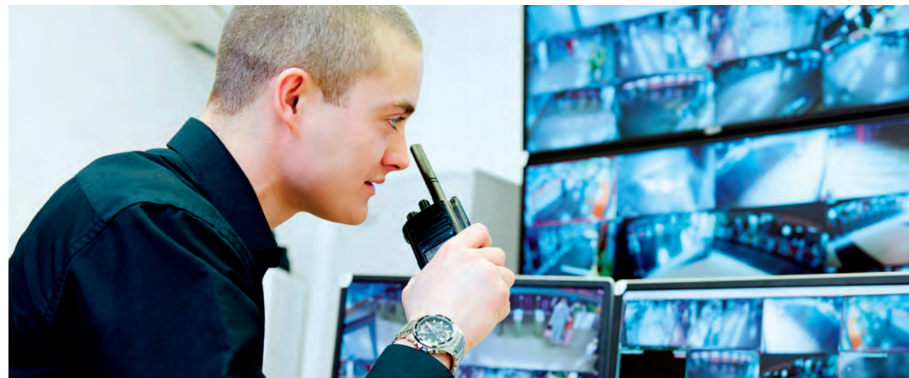
Expercité — The Expercité integrated automation system coordinates all existing equipment to manage urban services more efficiently.
