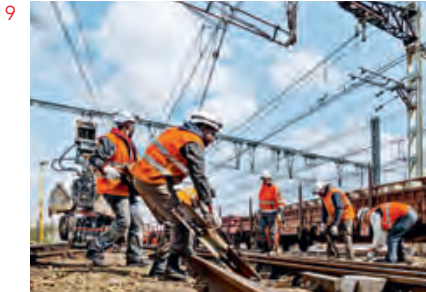
9 Replacing track equipment in Brétigny-sur-Orge.
