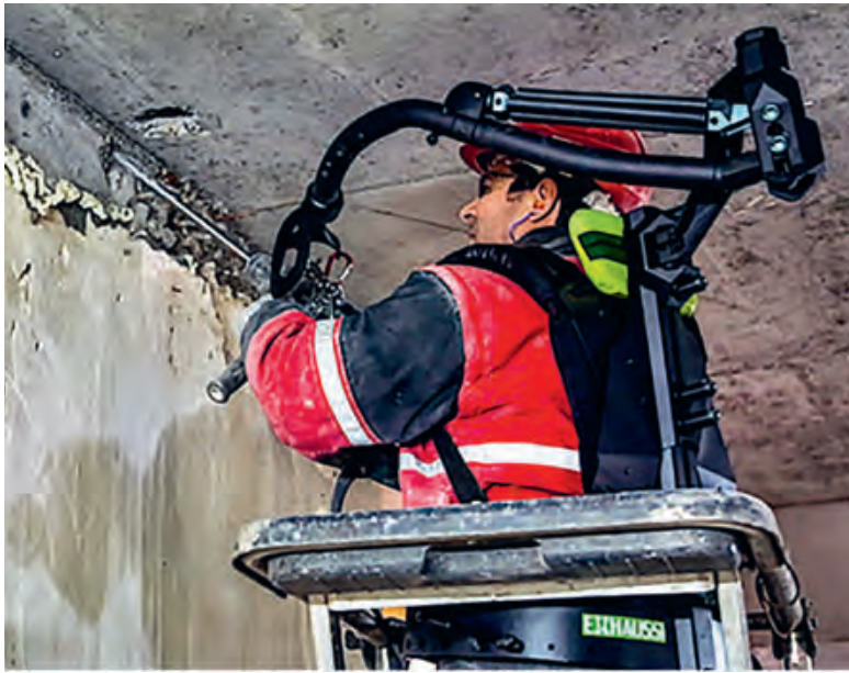
Testing an exoskeleton designed to reduce the risks associated with carrying tools and to facilitate movements, during work to renovate a listed mansion in Rue de Courcelles, Paris.
