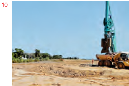
10 Foundations for the future Ariane 6 launch pad at the Guiana Space Centre in Kourou.
