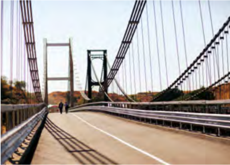
Kamoro (Madagascar) — Projects to build a new dual two-lane suspension bridge and renovate the ageing Eiffel bridge in Kamoro were completed in 2017.
