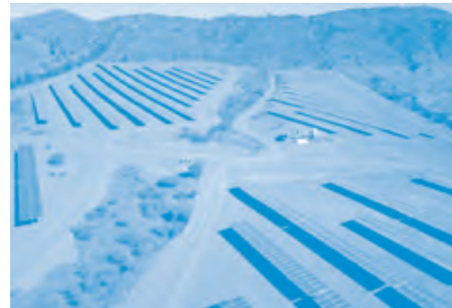
Marchihue VII photovoltaic plant © Eiffage Energía Chile
