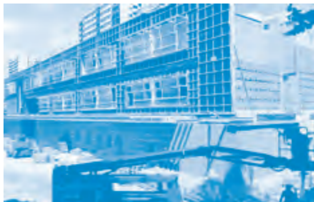
Construction of the Paul Langevin school complex in Fontenay-sous-Bois © Eiffage
